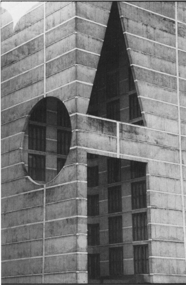
Fig. 30. Detail, office block, National Assembly, showing marble banding at five-foot intervals. Illustrates relation of banding to windows indoors, and the alternation of flat bands with projecting drip courses.
